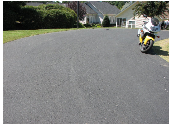
One cul-de-sac traffic circle showing uniform seal-coat application
