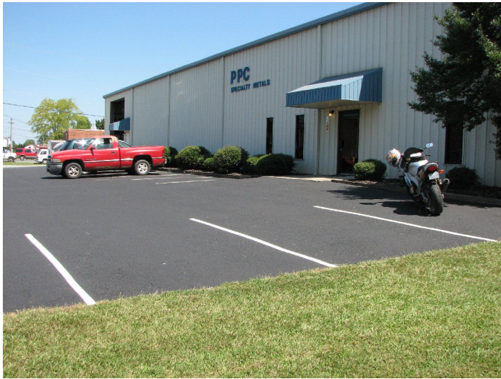
Uniform sealcoat application, clear striping
