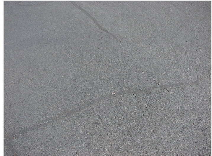
Cracks completely filled
