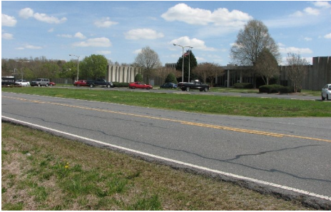
NC Highway 75 at Parkdale Mills in Mineral Springs
