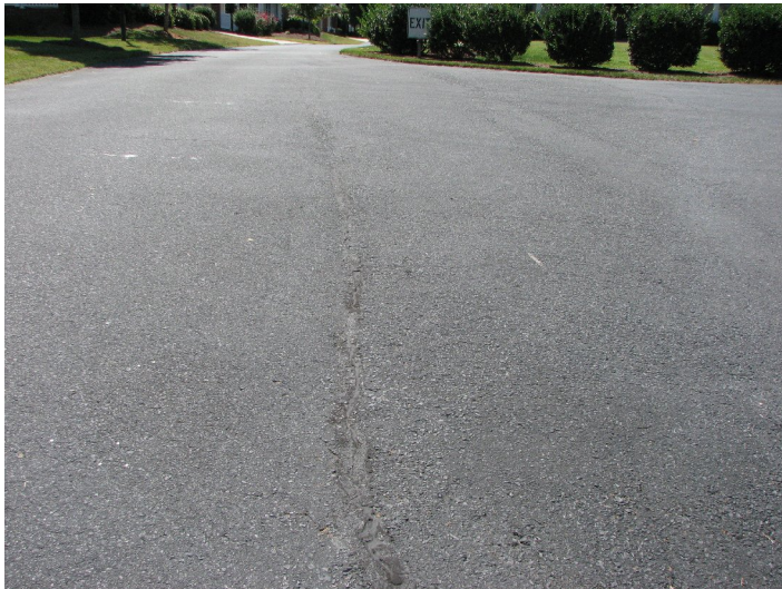
Road centerline joint/crack completely filled
